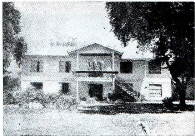
Girls' Dormitory Built in 1938, with Some Modifications.
